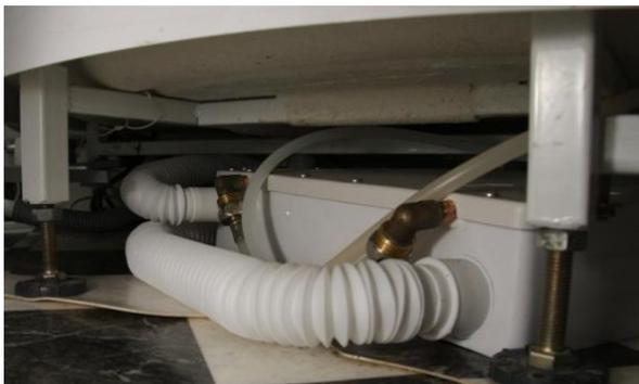
We recommend the use of a hair catcher. HeatSnagger will work even without any maintenance but we recommend to flush with hot water every second month to maintain a good efficiency rate.
